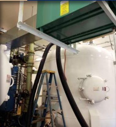
The District's Arsenic Removal Filter System
