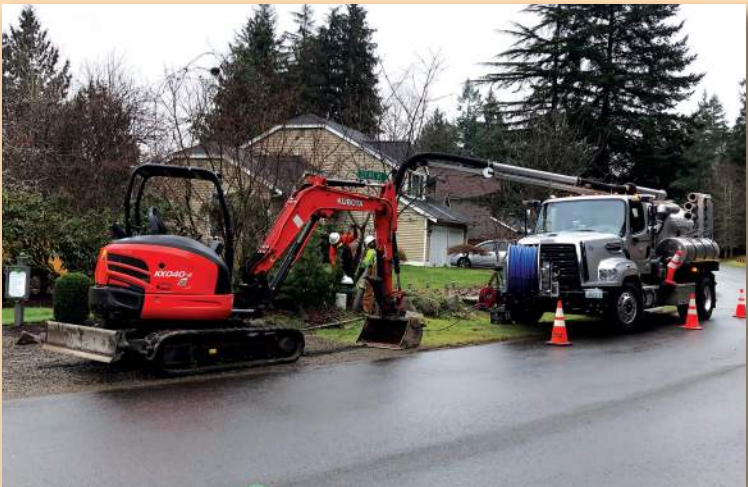
District staff replacing a fire hydrant.
