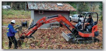
District staff preparing site before pouring concrete pad for a new well-field generator to ensure water supply.
