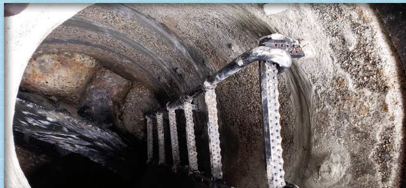
New manhole casting (top), ladder and joint grout (lower).
