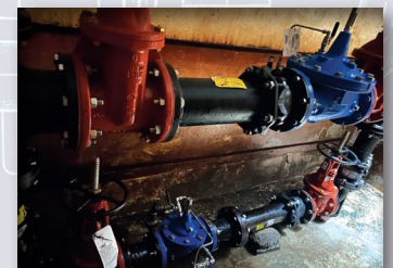
Newly rehabilitated pressure reducing station.
