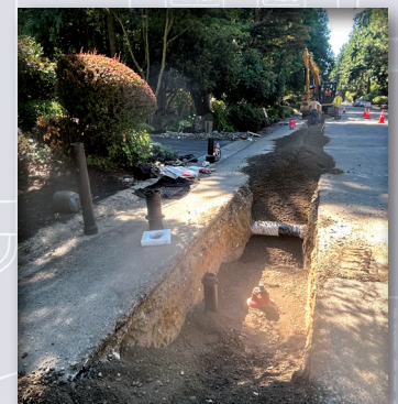
The AC pipe replacement project under construction.
